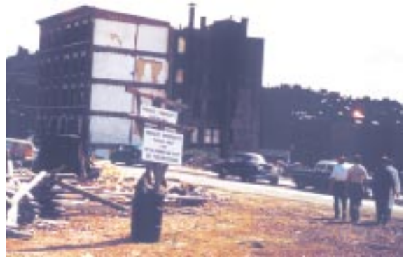
Figure 8: The Retina Foundation, 30 Staniford Street, in 1960
